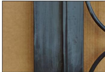
Inspect damaged area to be repaired. If the unit has deep gouges, they may have to be filled with Bondo, sanded flush, then finished.
